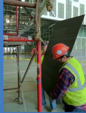
Moving Back-Buttered Half-Size Panel
