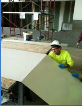
Snapping Panel After Scoring With Cutter
