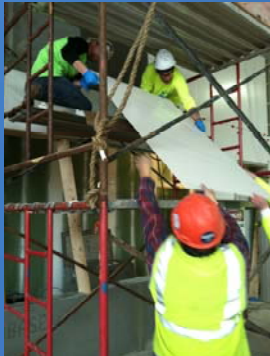
Lifting Back-Buttered Panel For Installation @ 17' AFF
