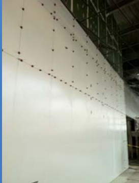
Leveling System Remains In Place For 24 Hours
