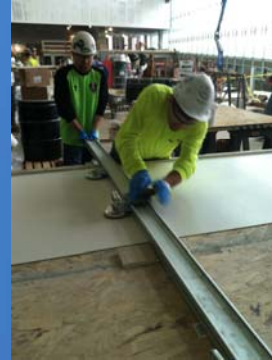
Scoring Panel To Cut Using 10' SIGMA 8E KERA CUT 128 Tile Cutter
